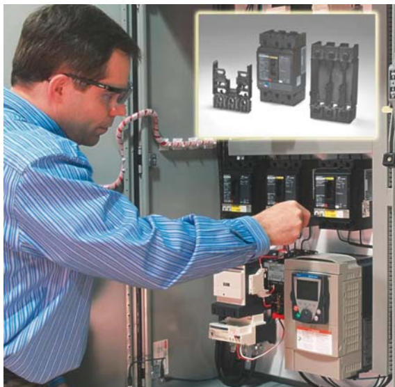
Fig 43. Polyamide has an excellent combination of good electrical properties, high operating temperatures, and flame-retardant capability (up to UL V-0 classification). The material is therefore used for electrical components such as fuses, circuit breakers, transformer housing, etc. Photo: DuPont
